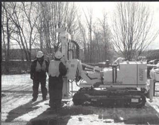
Our Brand New GeoProbe 6620DT Drill Rig
